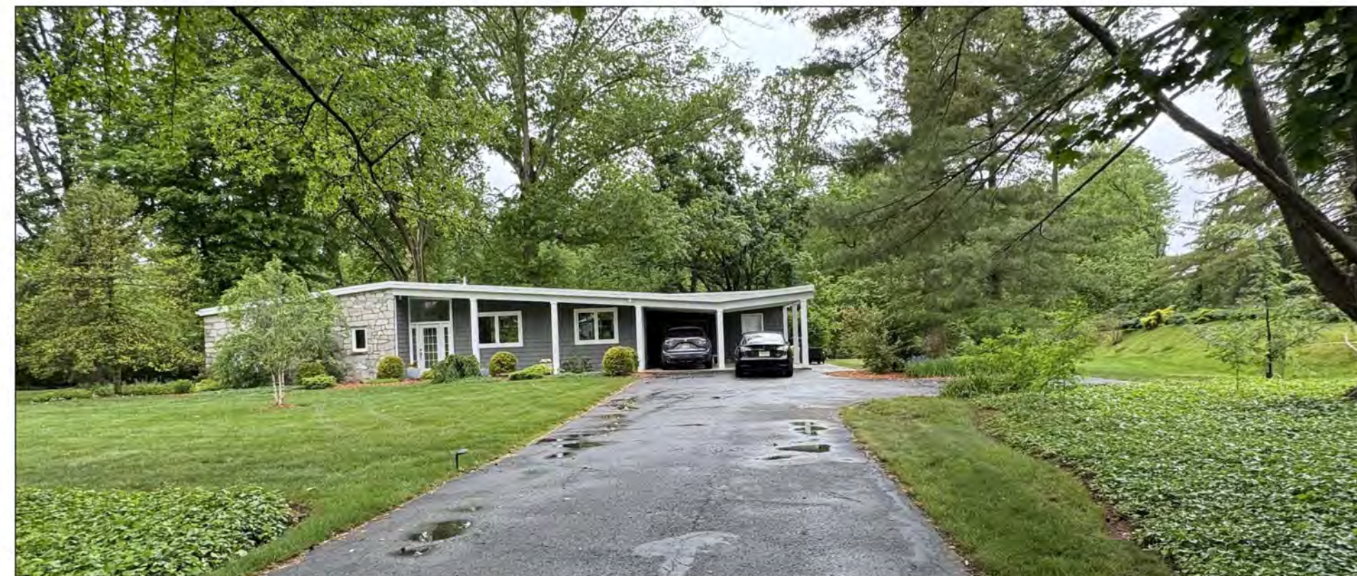
VIEW FROM DRIVEWAY TOWARDS FRONT OF HOUSE W/ RIGHT SIDE EXT. PARKING AREA/PROPOSED CARPORT
