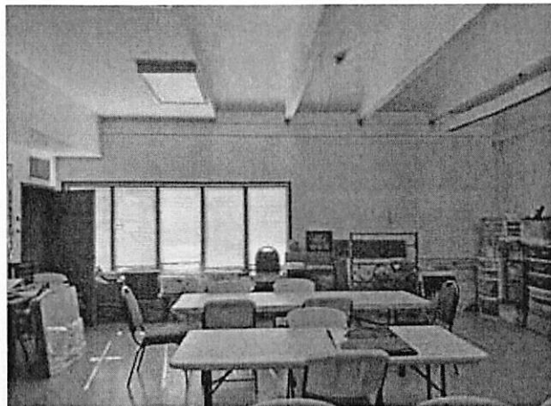
View of ceiling and window
