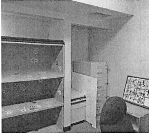
Plywood shelving and configuration of soffits and walls
