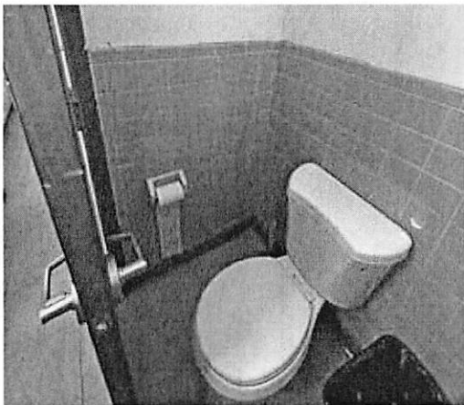
Existing toilet and accessories with door open
