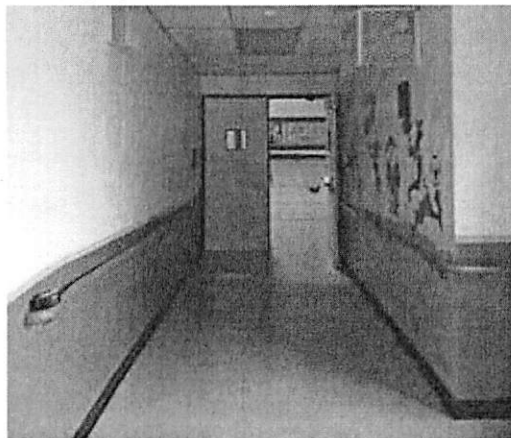
Ramp to gym
