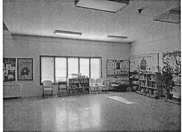
Existing window to remain
