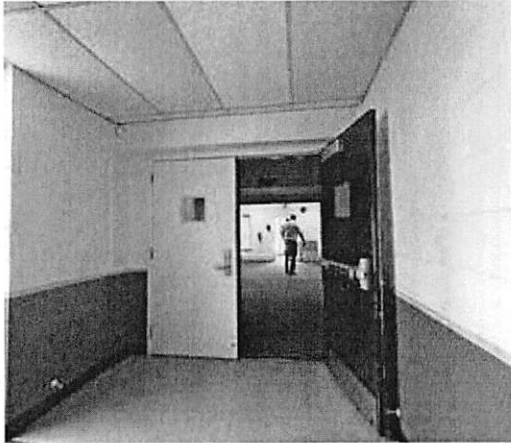
View from vestibule looking towards main building lobby
