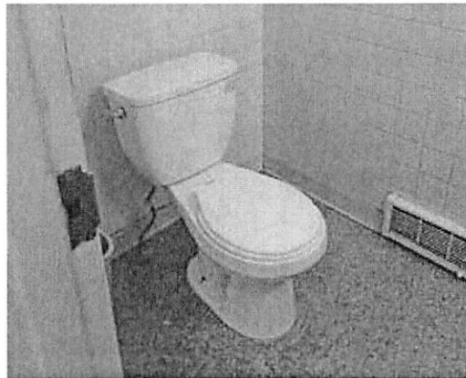
Men's toilet and existing baseboard heating
